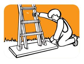
On soft ground use a wide board (6 inches width or more) to keep the ladder legs from sinking into the ground and slipping.
